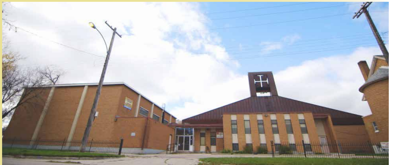
Gonzaga Middle School is set to open its doors in September, 2016.
